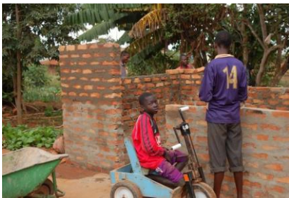
The chicken house under construction
